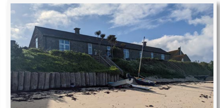
Bomb store building then (after the explosion) and now
