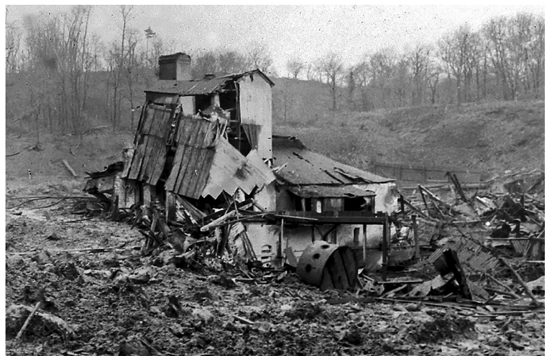
The gypsum works destroyed by the explosion and flood from the reservoir.
