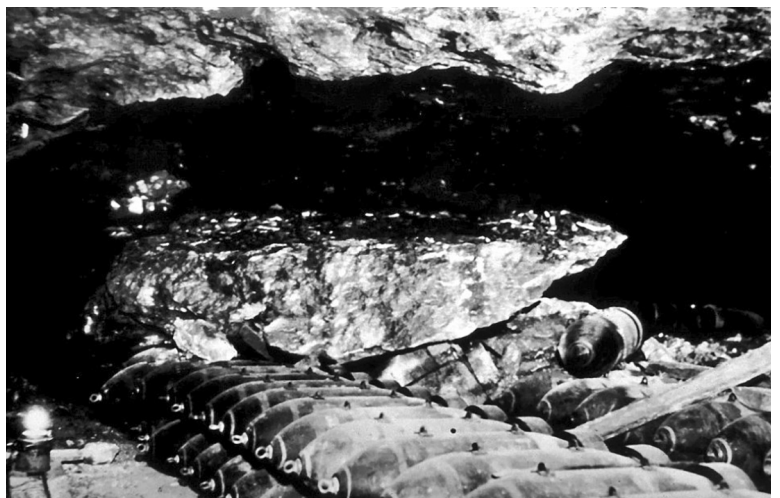
Roof collapsed onto aerial bombs
