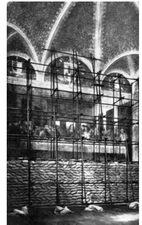
The construction of a protective wall saved Leonardo da Vinci's painting, The Last Supper . In 1943, a British bomb landed just ninety feet away, obliterating the roof of the refectory housing this masterpiece.
